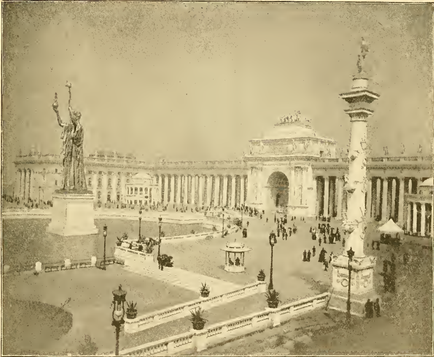
PERISTYLE, FROM THE AGRICULTURAL BUILDING.
